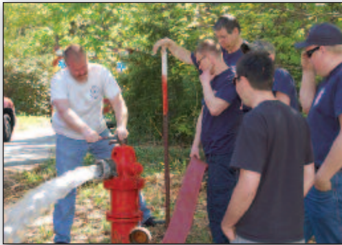
Class participants flow test a hydrant.
