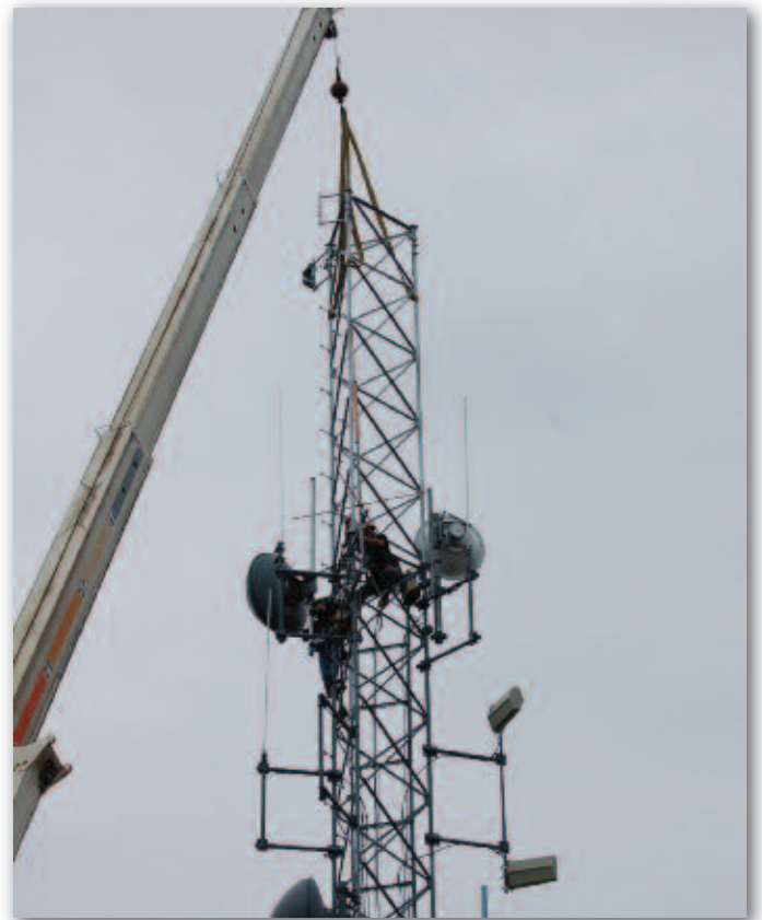
On April 3, 2011, the antenna tower at LRMFA had 20' added to the top to make room for the state to add microwave antennas. LRMFA's antennas and camera were moved up to limit interference.
