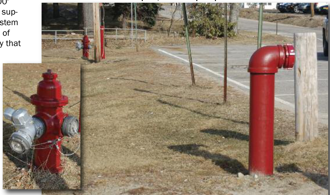
Below, left: Closeup of "push" hydrant where the hydrant system in the village begins. Below, at right is the dry hydrant that reaches out into Lake Winnepesaukee. The push hydrant is seen in the back of the photo, near the telephone pole.
